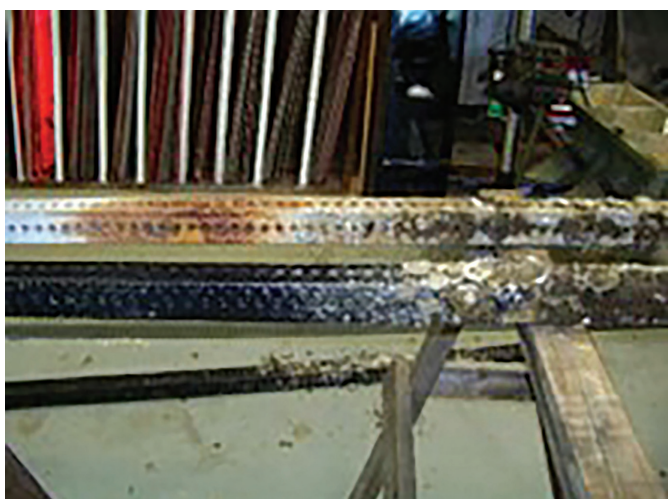
APC post and galvanized post after 13 months in the ocean.
